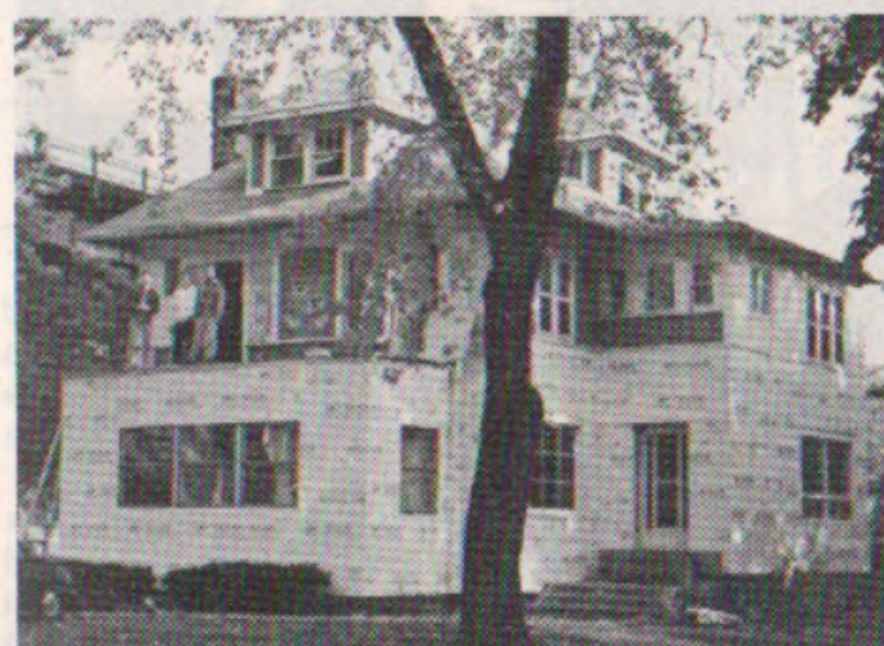
Insulation installation gives the Windsor Chapter house a temporary new look.
