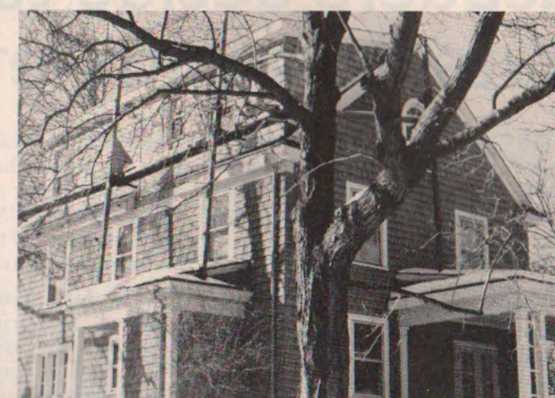
The full dormer to the third floor gives needed additional living space
