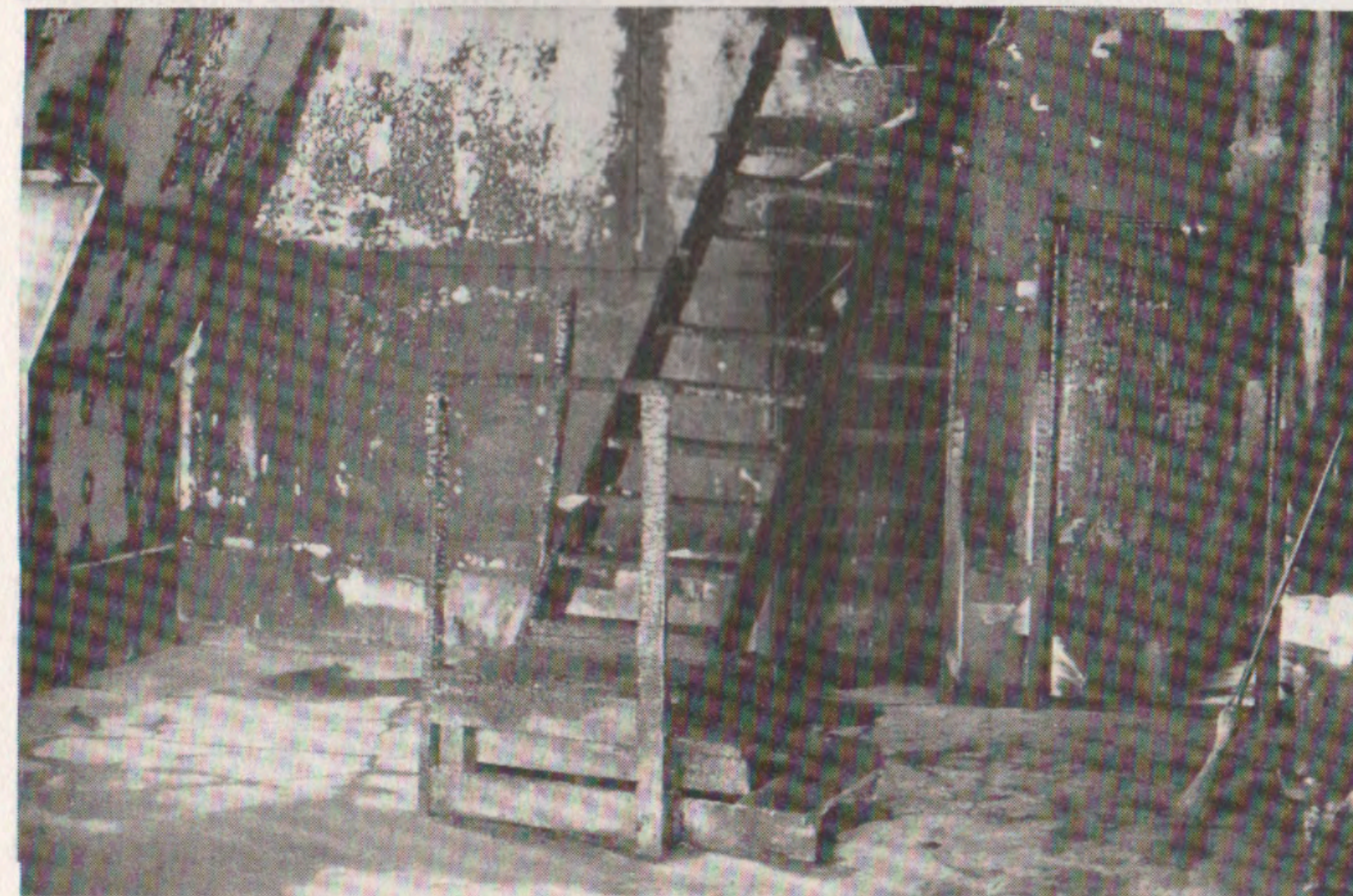
Upper left: Fire doors save the remainder of the house, preventing the fire spreading down to the lower floors. Left: Stairway from the dorm to the storage area.
