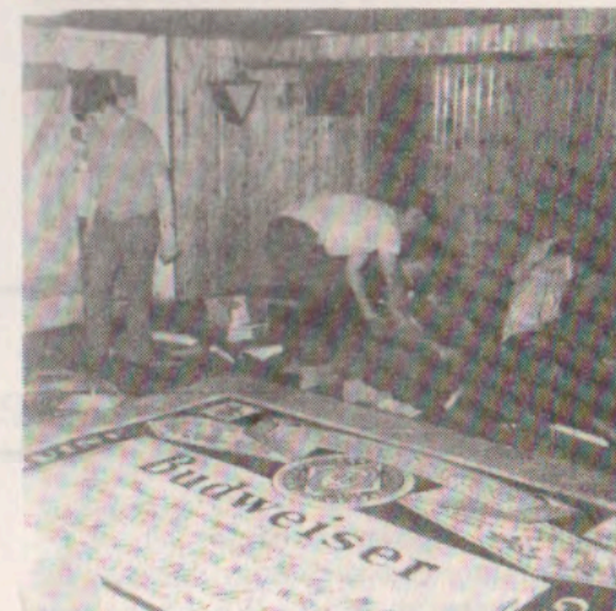
Some of the Tri-State Chapter brothers installing their new party room floor—Just like on TV. (Groovy)
