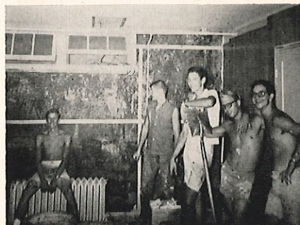
Members at work (?) during Work Week at Kansas State.
